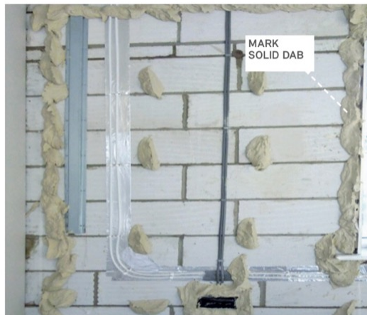
Builders Handbook Guidance Regarding Plasterboard Sealing
