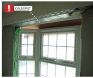
THICK FRAME AND POSTS INCREASES HEAT LOSS
